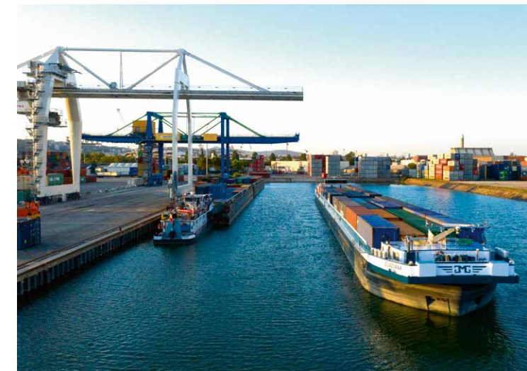
▲ The container and heavy cargo terminal at port de Lyon with its 2 travelling cranes.
