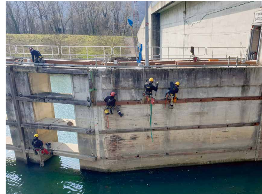
◀ Maintenance while navigation is stopped.
