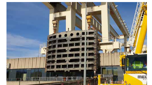
▲ Renovation of the downstream gate of turbine unit 6 of the Caderousse plant.
