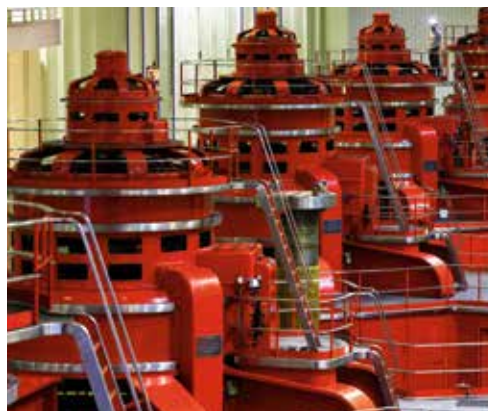
Engine room of the hydropower plant of Génissiat
