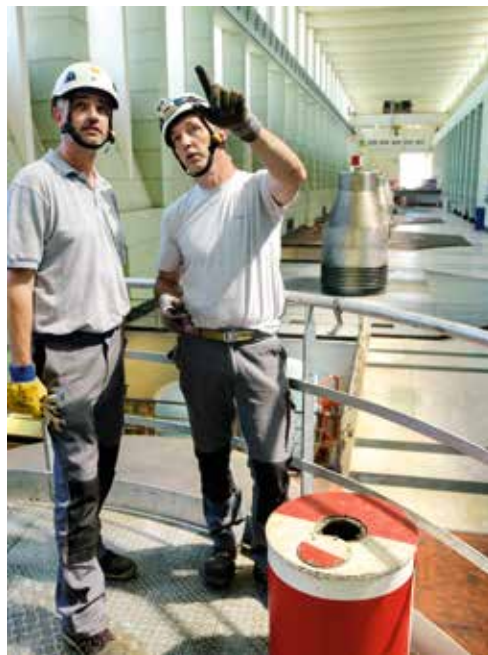
Operation in the machine room of Bourg-Lès-Valence
