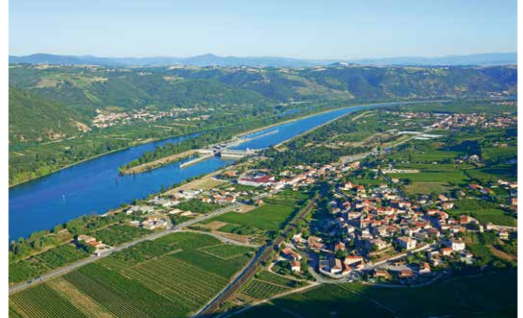
Aerial view of Saint-Vallier, the plant-lock of Gervans
