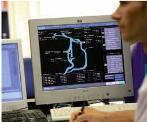
Control room of a hydropower plant
