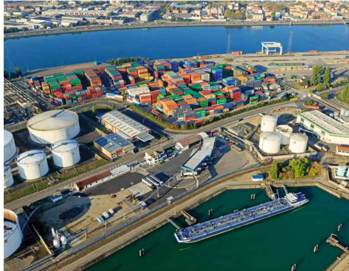
Aerial view of Port de Lyon Edouard Hériot
