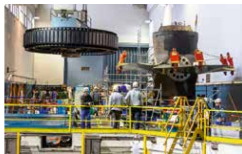
Renovation of turbine unit 1 at Logis-Neuf
