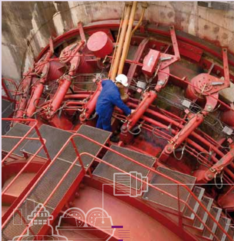
MAINTENANCE OF A PRODUCTION UNIT - CHAUTAGNE HYDROPOWER PLANT
