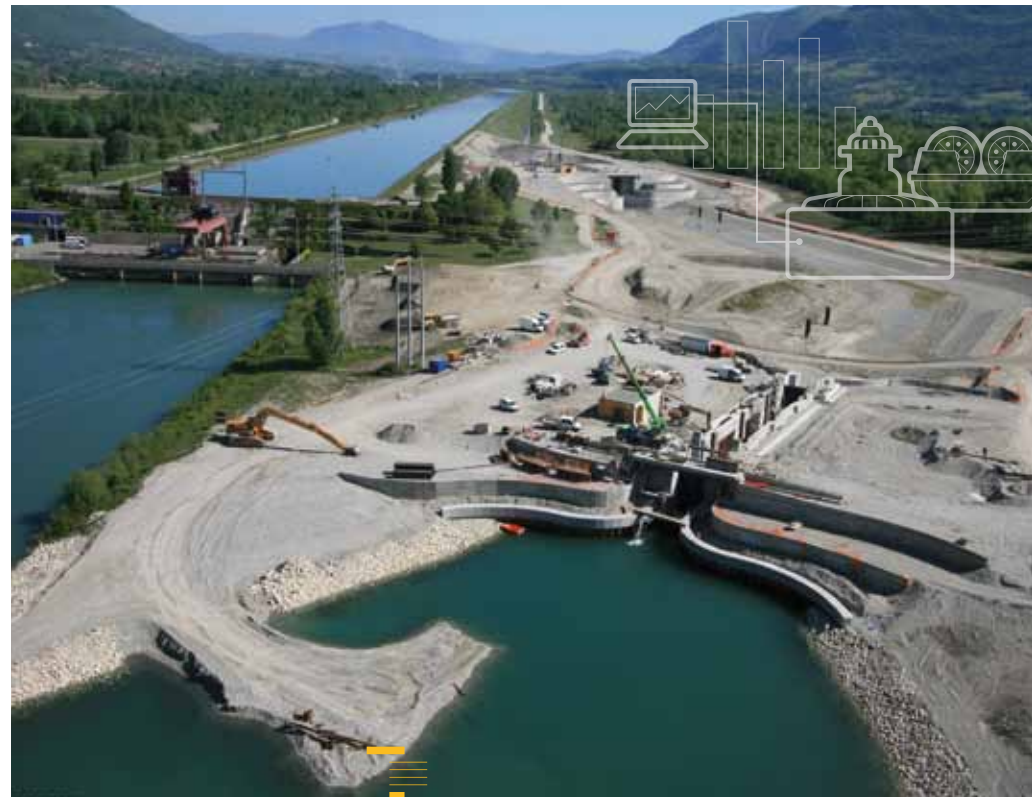
CHAUTAGNE: THE ANGLEFORT HYDROPOWER PLANT AND THE CONSTRUCTION OF A LOCK
