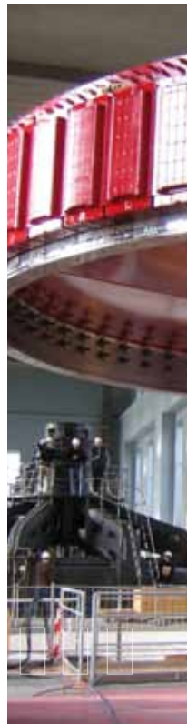
ASSEMBLING A NEW ROTOR AT CHANCY-POUGNY (SWITZERLAND)
