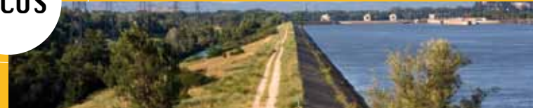
DIKES ERECTED ON THE RHÔNE
